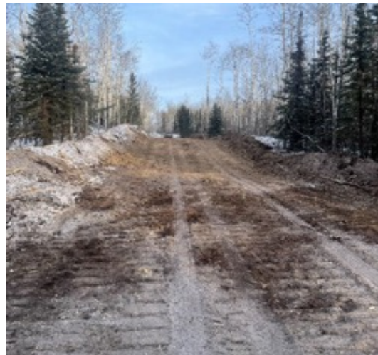
Finished Product of dozer at KP 143.3, Mulch on left and side slope material on right.
