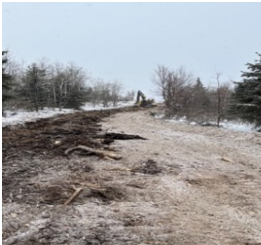
Excavator cutting side slope at 134.2
