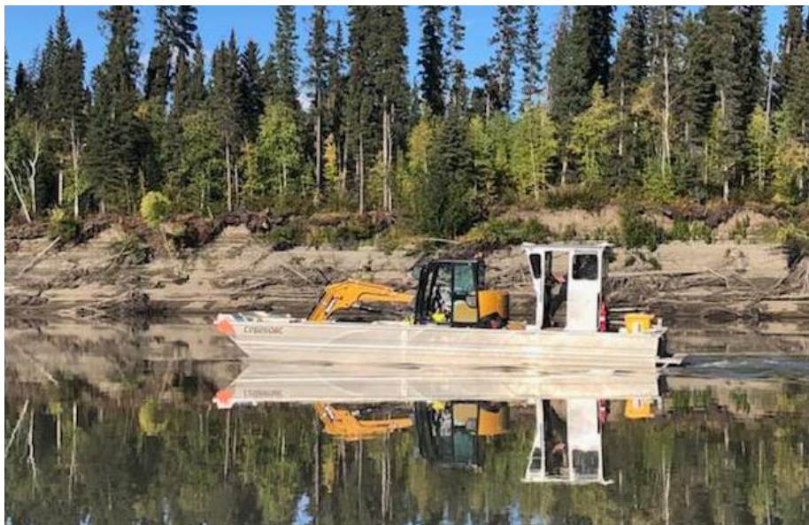
The barge crossing of the excavator across the Liard River
